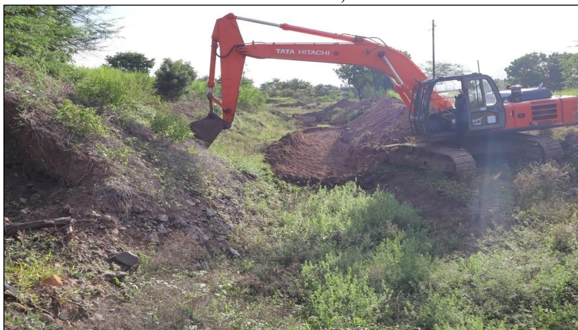
Decrease in water storage capacity of water stream due to silting At- Lawandewasti, khor
